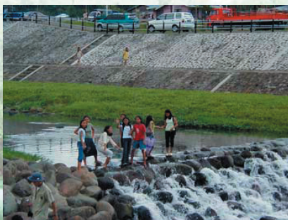
Flood Mitigation in Ormoc City, Philippines
