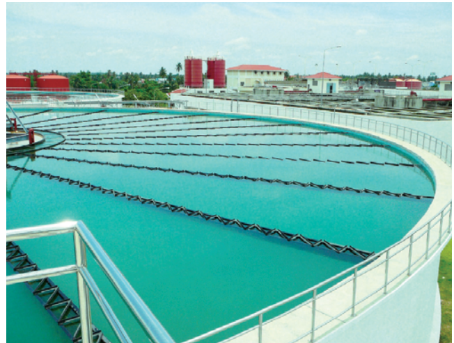
Maha Sawat Water Treatment Plant Solid Contact Clarifier 210,000 m 3 /day, 63m in diameter Manufacturers proposed design
