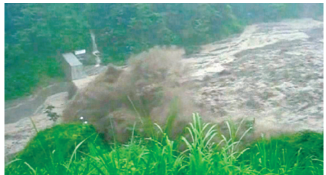
Debris flow attacking the New Sabo Dam on Feb. 16, 2007
