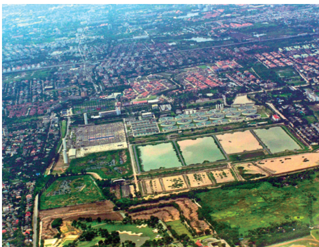
Bang Khen Water Treatment Plant
