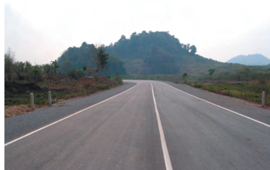
Northern Economic Corridor Construction Project Lao PDR
